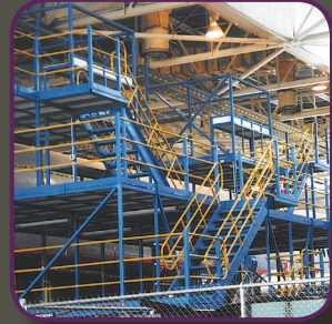
Custom designed access platform
